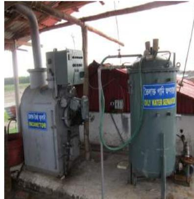
(c) Incinerator and oil/water separator
