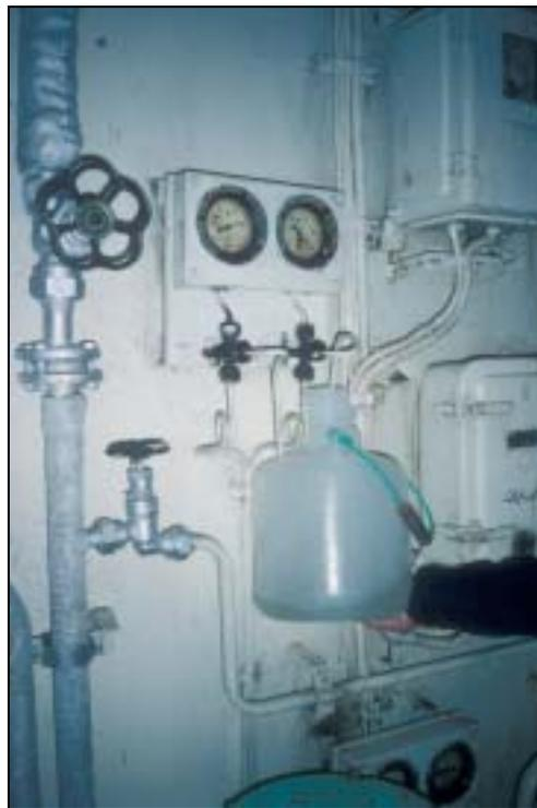
**Figure 1f.** Collection of samples from bleed valve in a ship's engine room.
