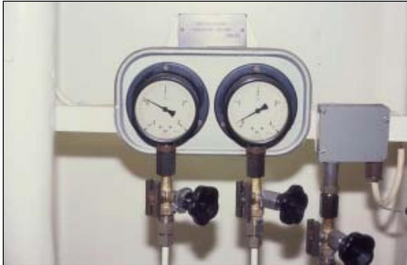
**Figure 4.** Pressure meter of ships ballast water pump.
