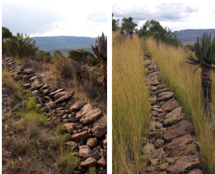
Stone lines constructed at a monitoring point at Ha Sekhonyana and regeneration of grass on the trapped soil at the same spot (five months after stone lines building and 12 months later) © ORASECOM
