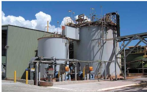
In mid-2011, a tailings paste plant was commissioned, which removes significant portions of the coarser content of the tailings discharge. Cement is then added to the coarser solids and the “paste” is disposed in the underground mine, resulting in about an 8% less solids in the tailings discharge.
