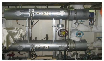
Figure 7.4 – Typical fuel oil heaters
