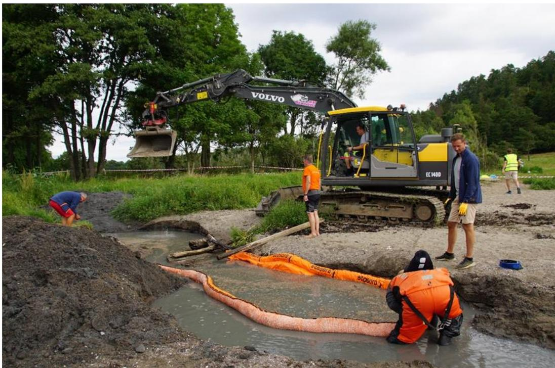
**Figure 24:** Containment and recovery using natural stream. Source: NCA
