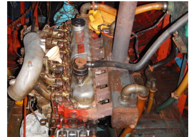
Diesel Main Engine
